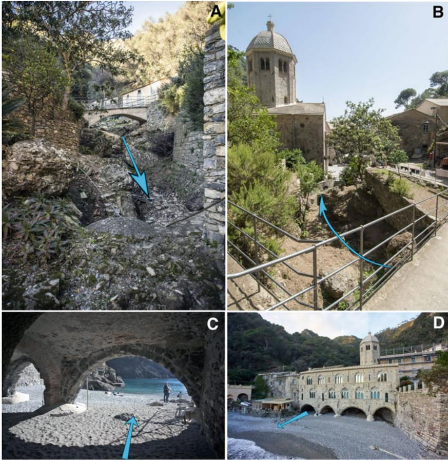
**Fig. 36.3** **a** The stream approaching the culvert running beneath the Abbey; **b** the culvert inlet; **c** the culvert outlet the beach; **d** view of the Abbey with the culvert outlet
