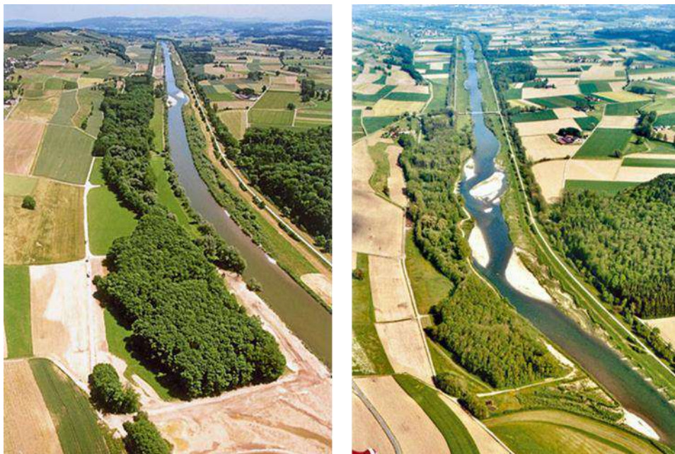
Figure 8-1 Thur river at Niederneunforn. Left panel: before restoration started in 2002. Right panel: after restoration in 2008. (© BHAtteam, Frauenfeld)
