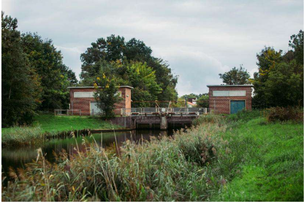
Figure 7-7 Lock and pumping station i river Egå near the Bay of Aarhus
