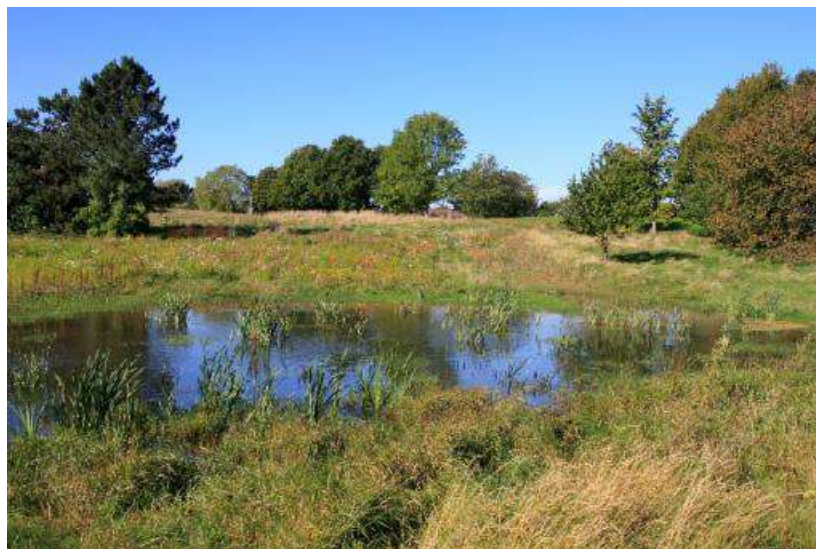
Figure 7-4 Green surface to a grey solution - a huge pipe is hidden behind the 'amphi-theatre'
