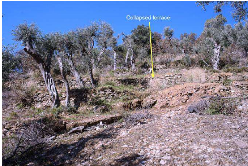
Figure 4-4 Pilot area – Vallone dei Fontanini: collapsed man made terraces.
