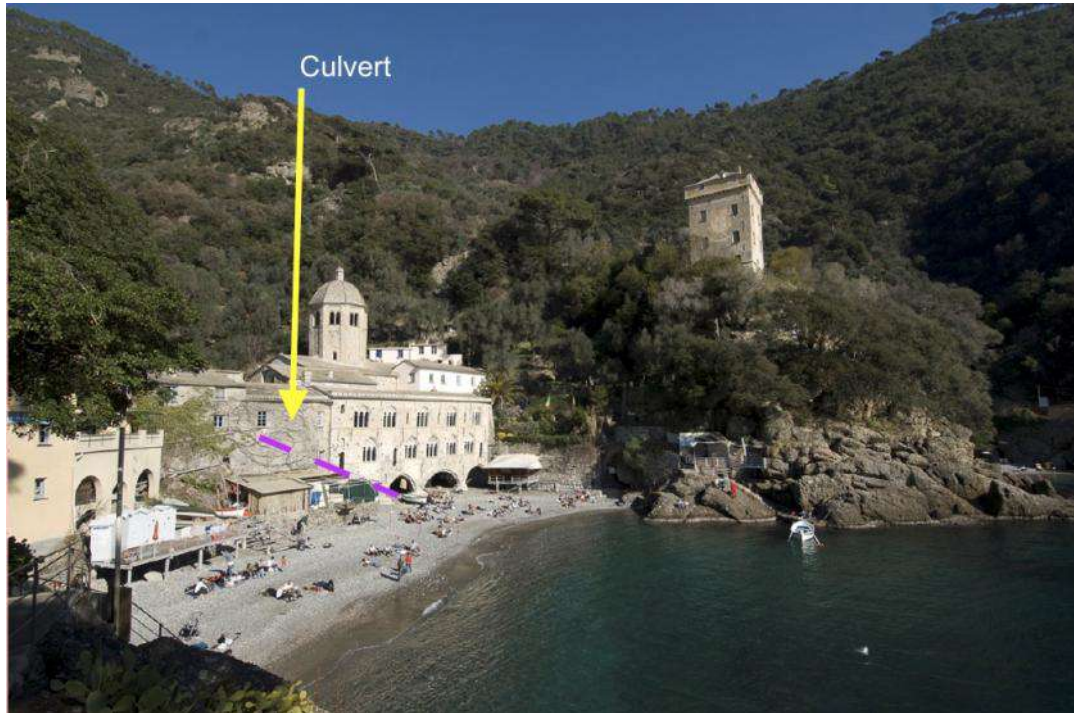
Figure 4-2 Pilot area – San Fruttuoso Abbey (X century) and the underlying culvert.
