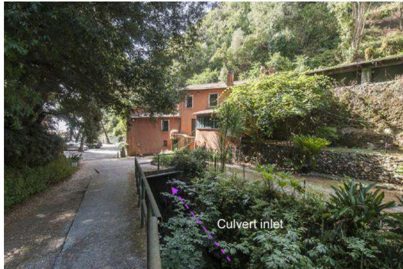
Figure 4-6: Pilot area – Paraggi culvert inlet.
