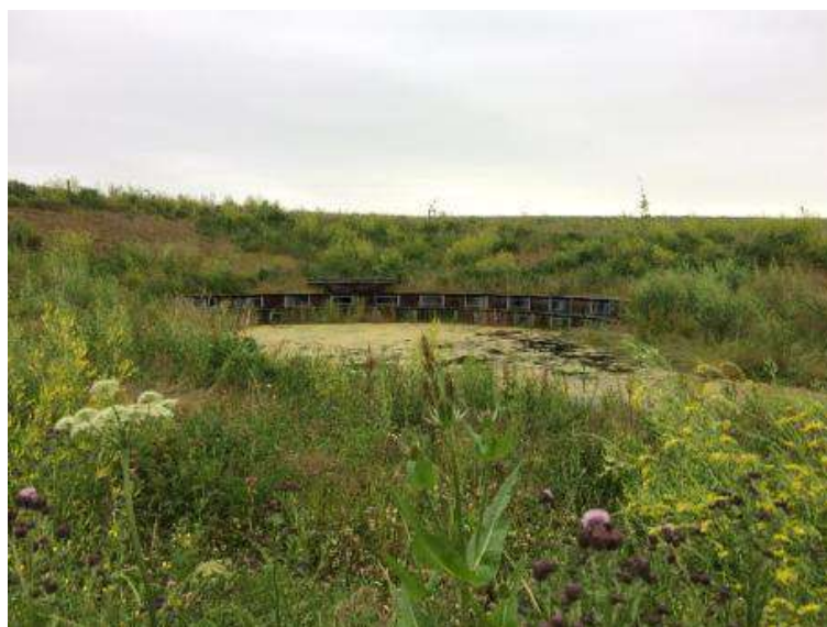
Figure 7-3 Green surface to a grey solution - a huge pipe is hidden behind the 'amphi-theatre'
