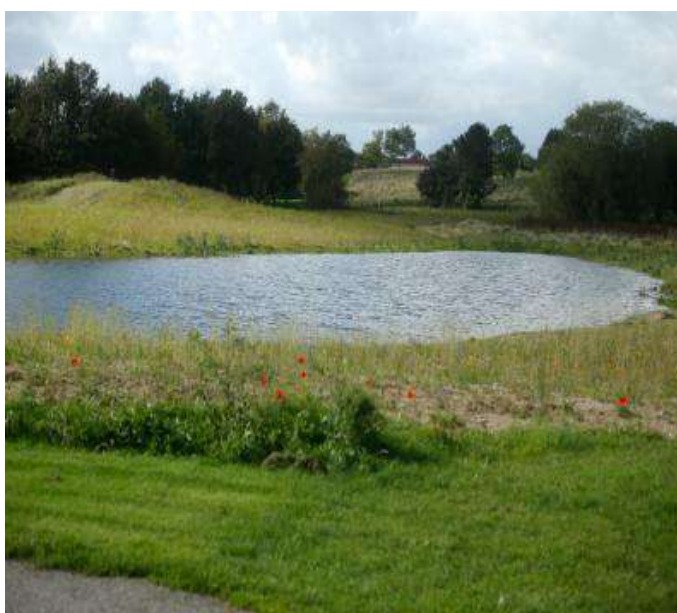
Figure 7-11 Green basin in Lystrup
