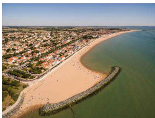
Figure 10-2 Protection wall in Les Boucholeurs
