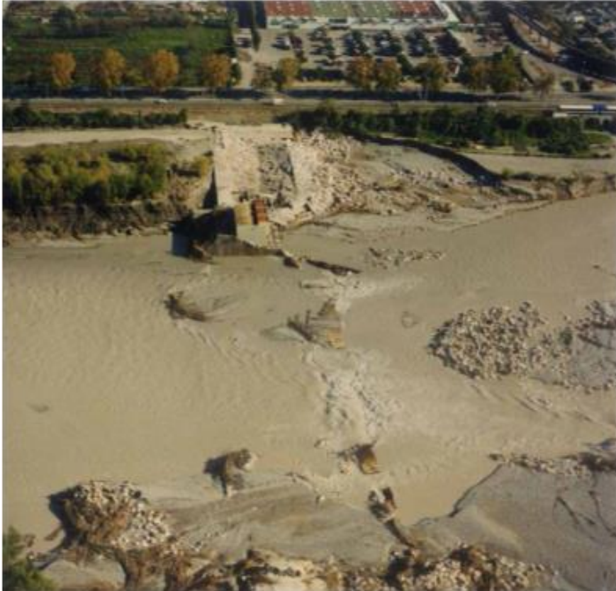
Figure 9-3 An example of the weir 4 after the event 1994.
