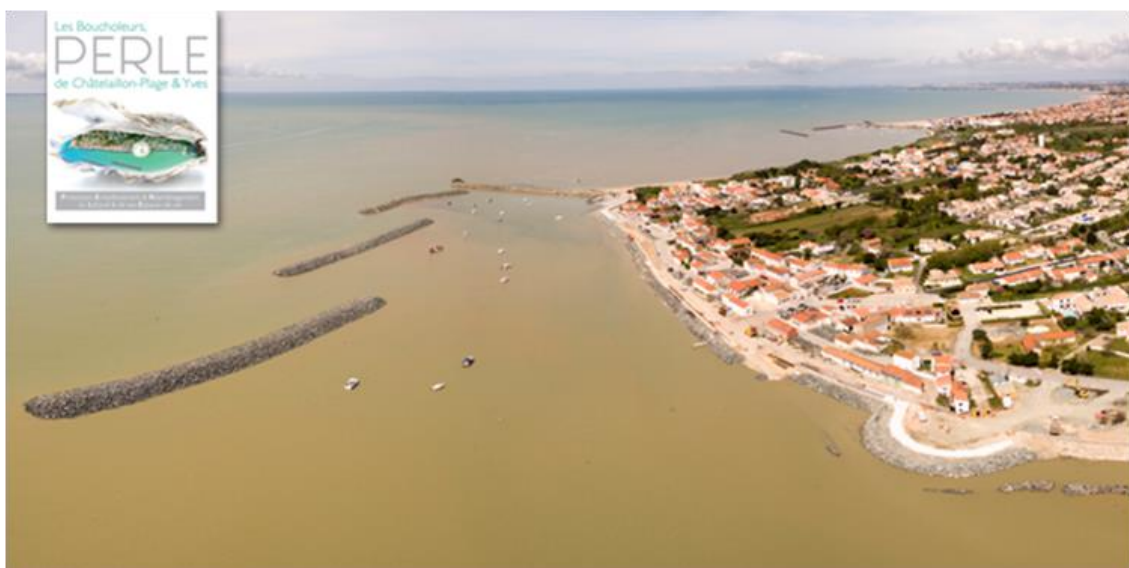
Figure 10-4 Breakwater structures located in the ocean close to the beach
