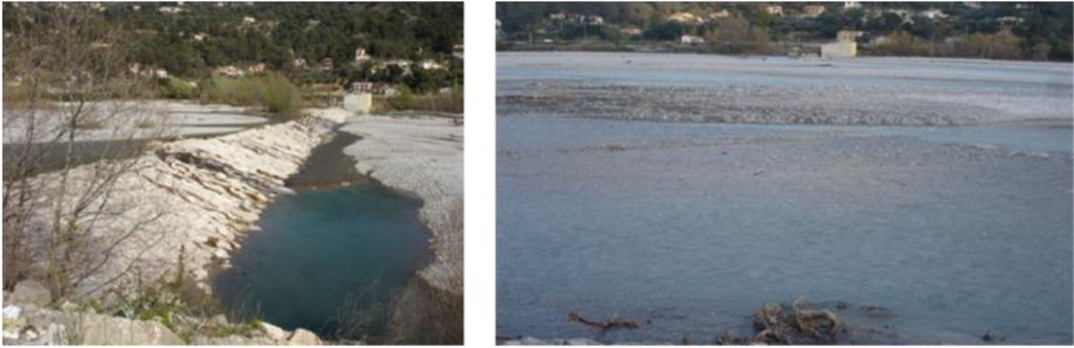
Figure 9-6 Effects on the weir 9, 2 years after intervention
