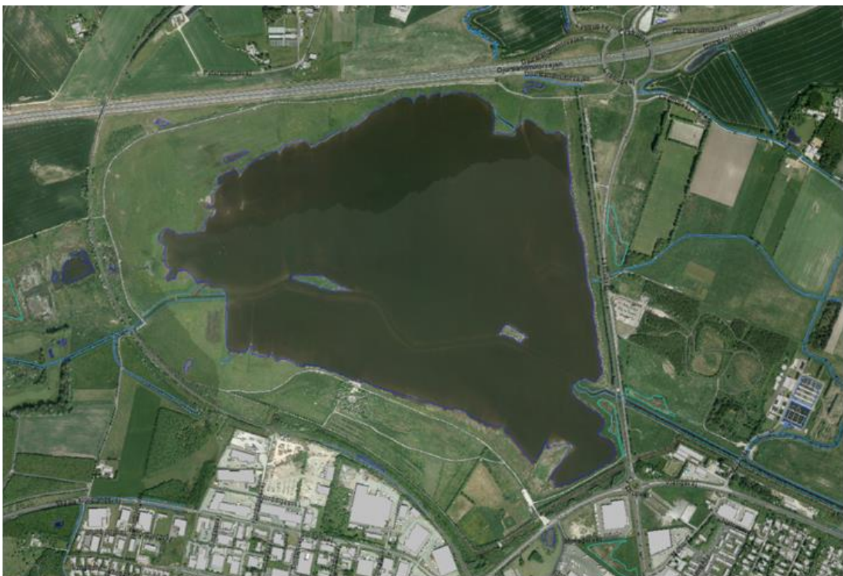
Figure 7-11 Project area after construction Lake Ega
