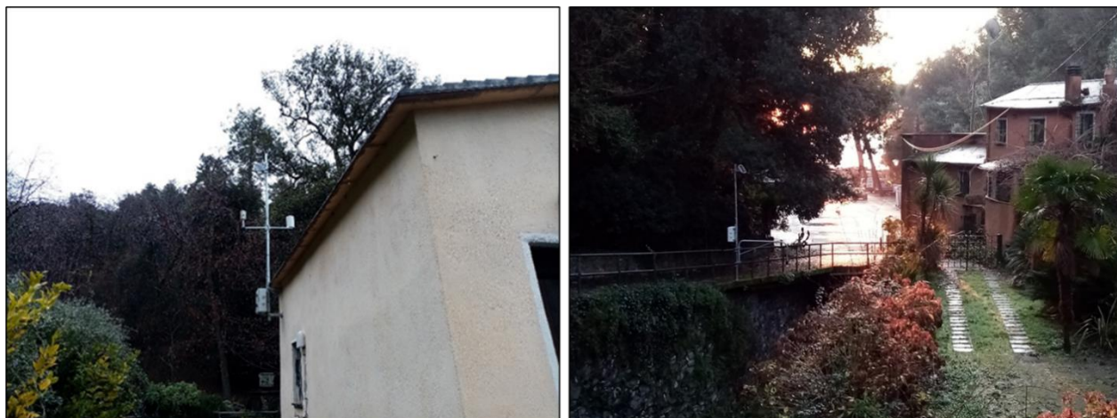
Figure 6-4 Installed weather stations in the Portofino Park
