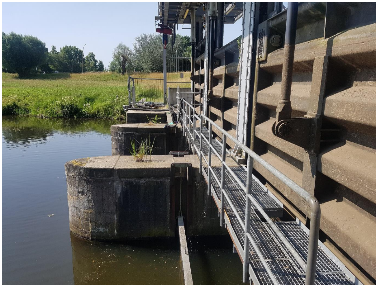
Figure 3-6 Inlets of the culverts of Tatenberg Sluice
