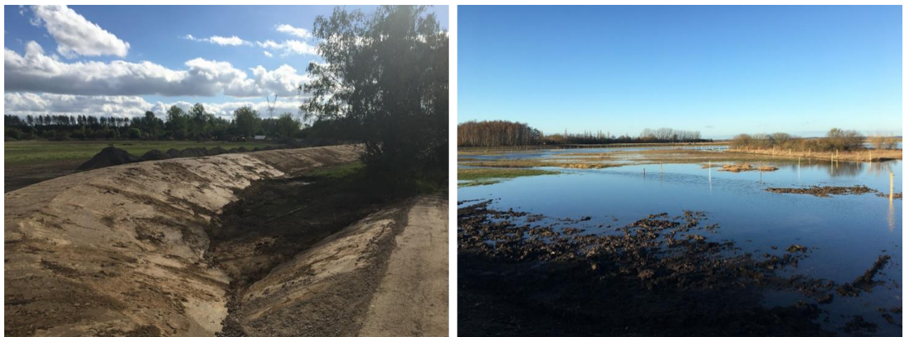
Figure 4-6 Left: new dike withdrawn from the coast. Right: land left on the seaside for natural succession.
