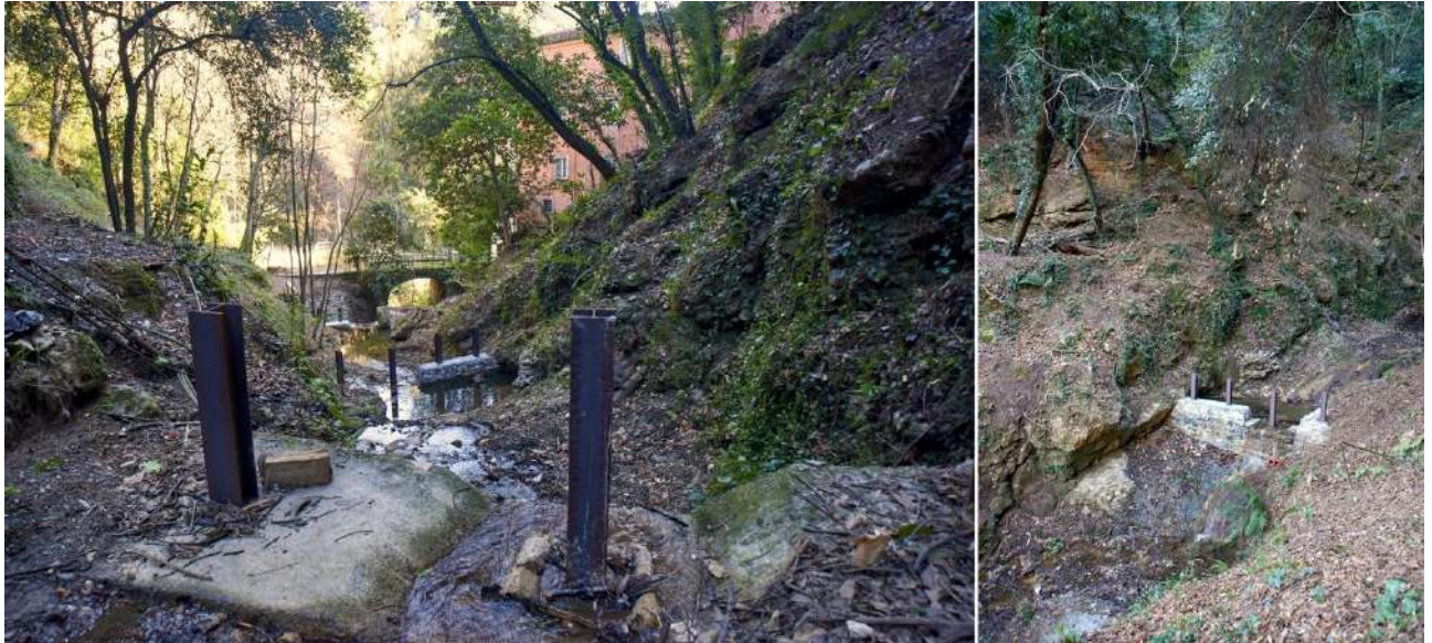
Figure 41 The floating transport selective weirs at the point 3a ( Error! Reference source not found. ) on the left, and stone and selective weir at the point 3b, on the right.
