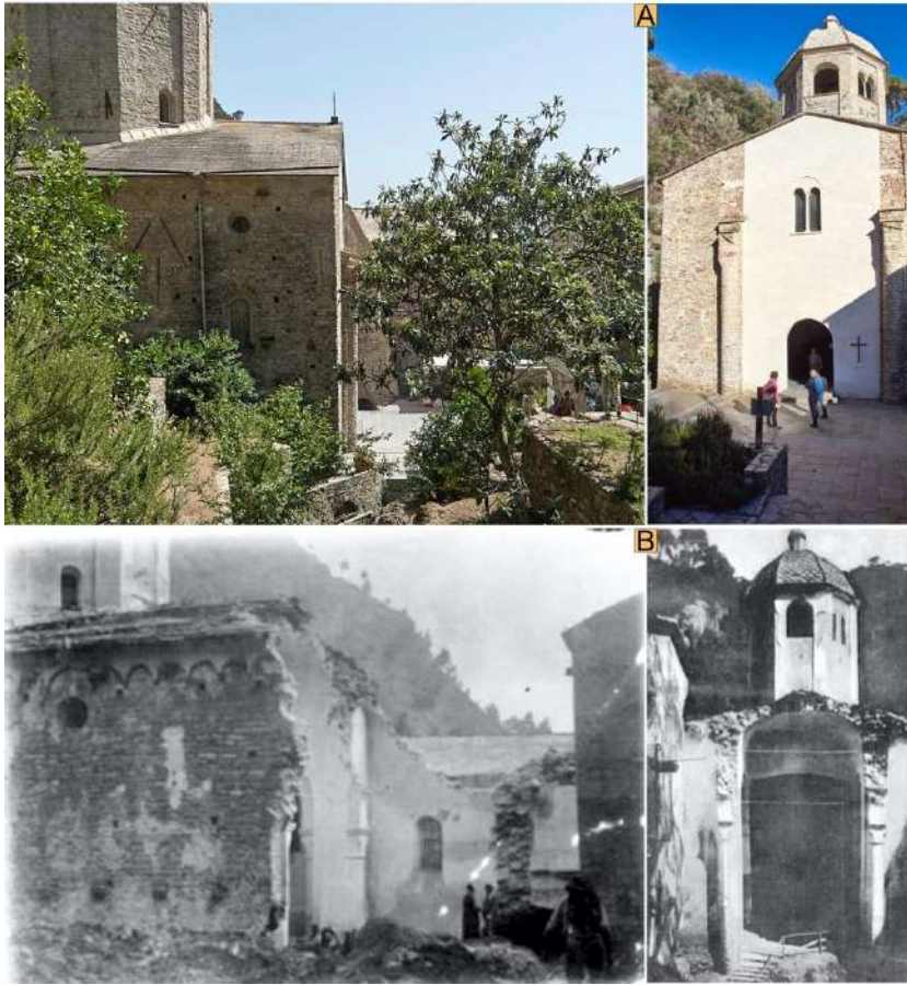
Figure 32 A comparison of the ancient abbey in San Fruttuoso as it appears nowadays (A) and as it was after the partial collapse in 1915 (B). (Paliaga et al, 2022a).
