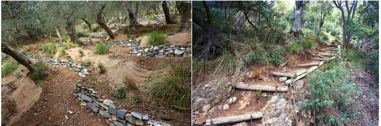
Figure 39 NBS measures in San Fruttuoso Bay: on the left terraces' recovery and Mediterranean scrub re-vegetation; on the right, trail maintenance with bioengineering techniques.
