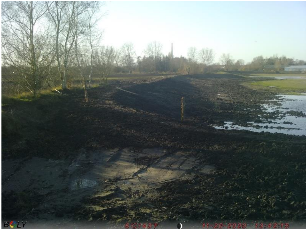
Figure 2: From the end of construction.
