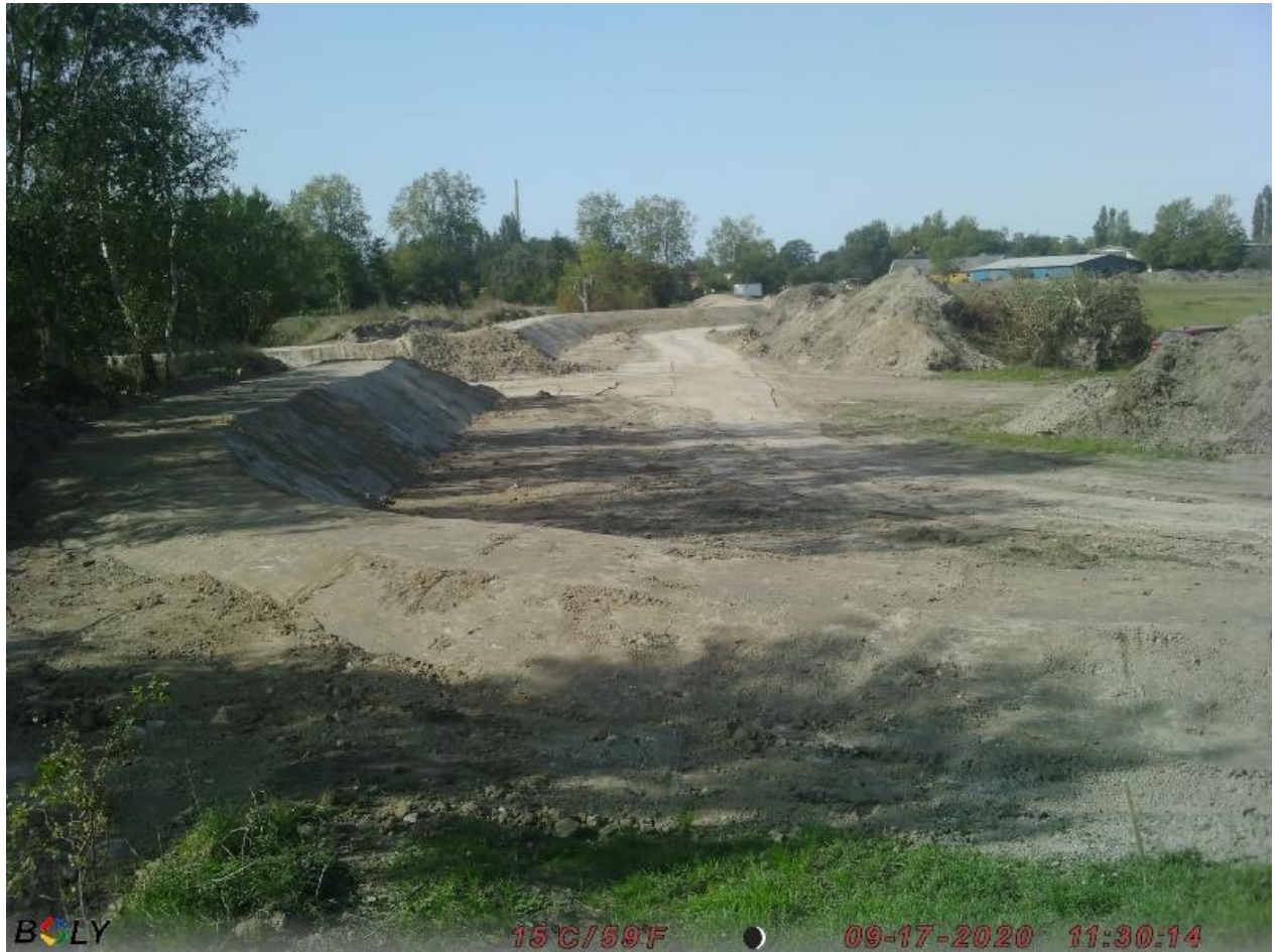
Figure 1: Picture from photo point from the beginning of construction.
