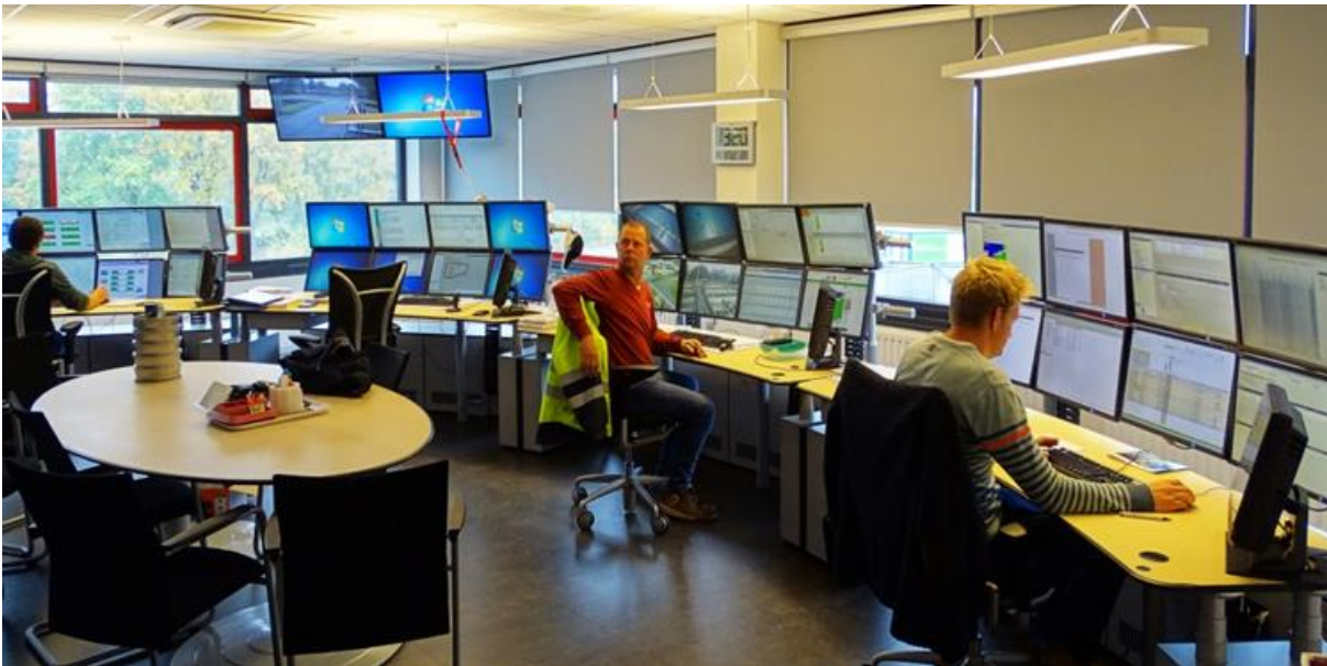
Figure 3. An example of a central control room that uses TeleControlNet
